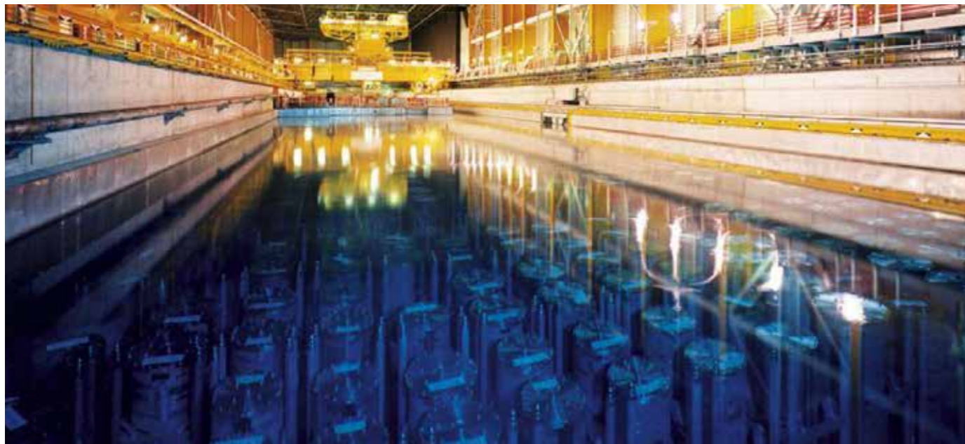
Spent nuclear fuel is to be held in carefully controlled storage ponds for many decades, until final geological disposal. NNL's work secures our understanding of how fuel will behave in such conditions, underpinning the decisions on how to manage fuel.
