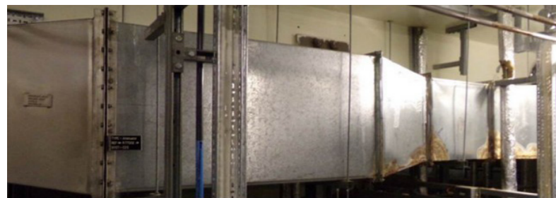
Central Laboratory C2 Duct repairs (before [left] and after [right])
